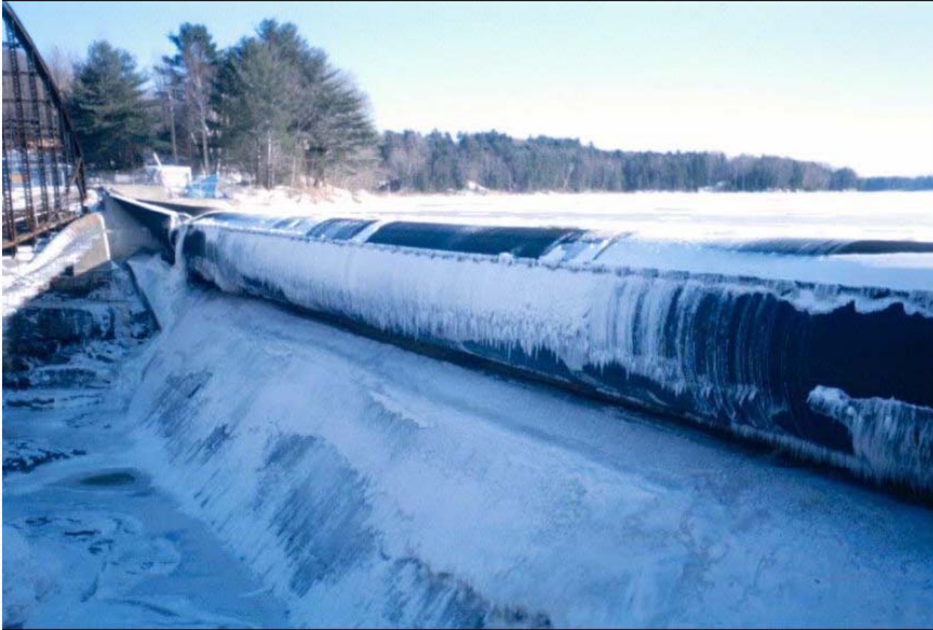
Şişme savak, Mississquoi River, Highgate Falls, Vermont, USA
